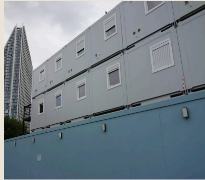
Portable Office Cabins
